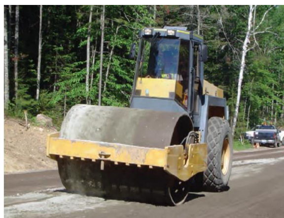
Figure 1 Rolling of Cement Treated Granular Layer II.LITRATURE REVIEW
